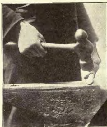
FIG. 42. FIRST STEP IN SHAPING A SCARF.
